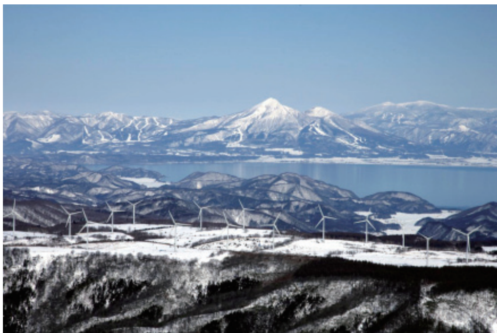
Kooriyama-Nunobiki Wind Farm of J-POWER in Fukushima prefecture ( Copyright(C) 2012 J-POWER All rights reserved)
