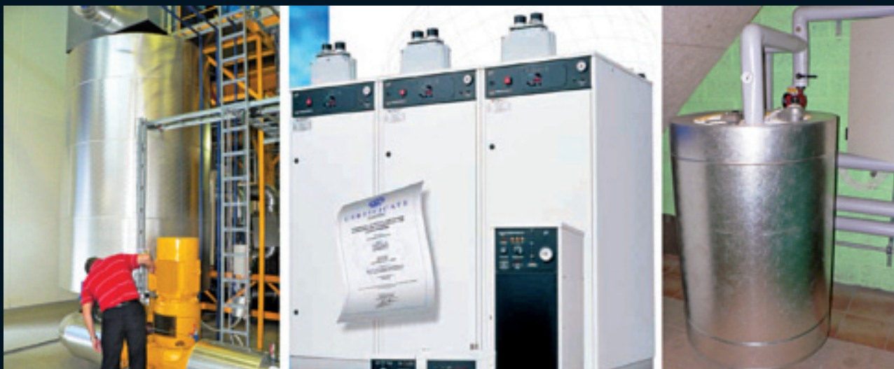
Figure 8 Three sizes and types of electric boilers for power down regulation. 20 MW, 10 kV (left); 3 – 300 kW, 400 V (middle); 45 kW, 400 V (right) (Nordic Folkecenter for Renewable Energy)
