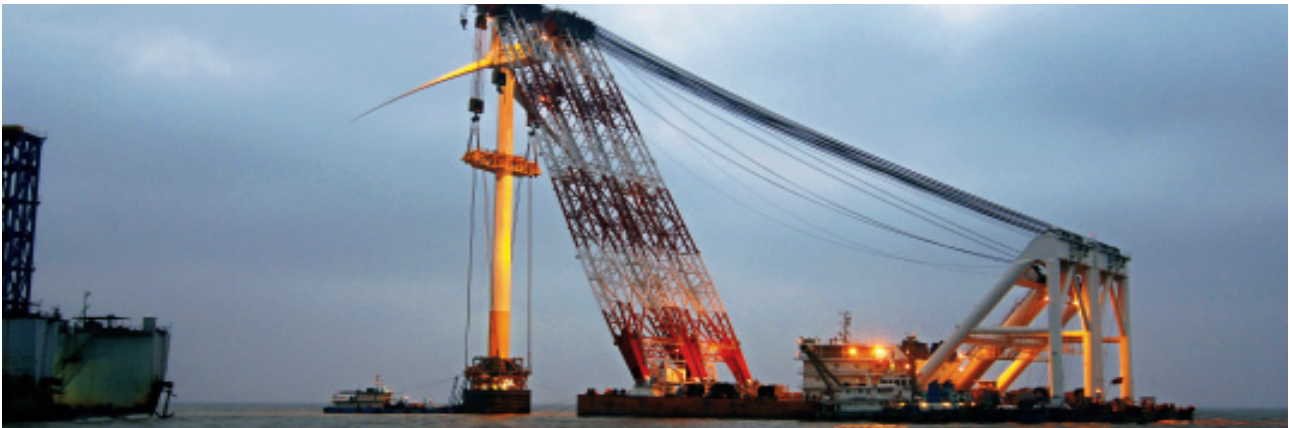
Figure 2 China's First Offshore Wind Farm (102MW) Constructed Near Donghai Bridge in Shanghai in 2009 (Source: Sinovel)
