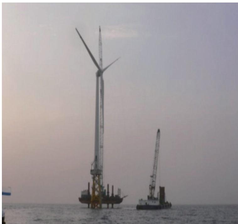
Figure 6 2MW OWT in Weoljung Offshore Wind farm in Jeju
