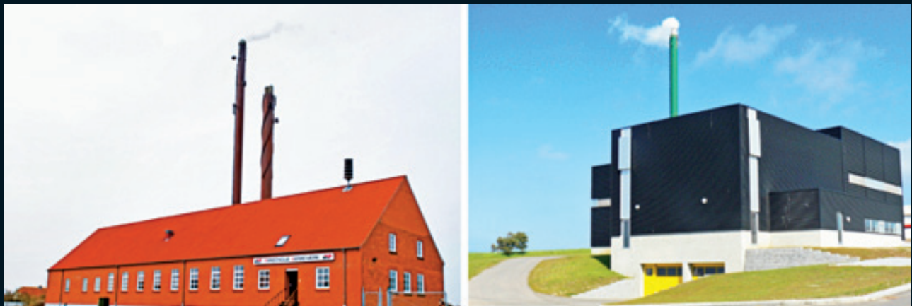
Figure 10 Hanstholm (left) and Hurup (right) district heating plants without CHP. Both are located in regions with high density of wind power. Hanstholm has installed 12 MW electric boiler to substitute the present fuels with excess power from local wind energy (Nordic Folkecenter for Renewable Energy)
